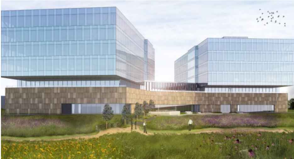
Reinsurance Group of America began construction on its 400,000 square foot headquarters.
