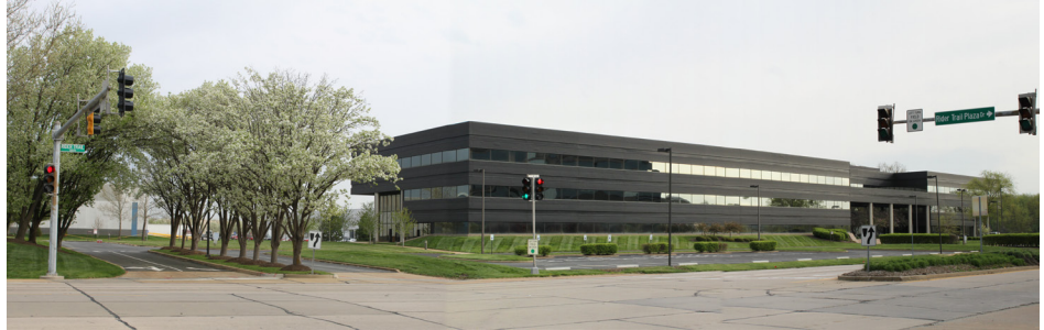
U.S. Bank moved into 46,000 square feet of space at 3301 South Rider Trail.
